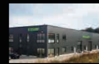
Germany Aachen R&D Center and Technical Center
